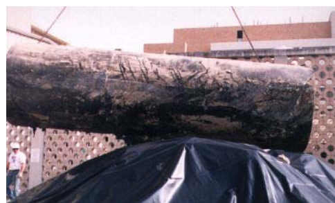
↑ 20,000 Gallon UST Being Removed from International Paper Facility in San Antonio, TX.
