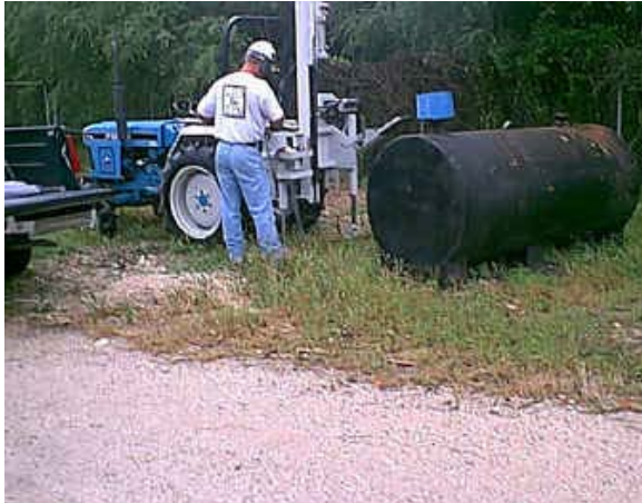
↑ Tractor Mounted Geo-Probe® Rig at San Antonio, TX.
