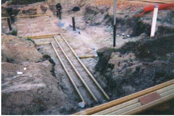
↑Fiberglass Pipe Installation at Exxon Station in Vanderbilt, TX.
